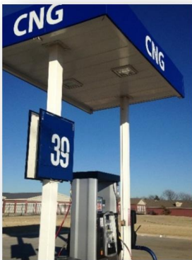
The Compressed Natural Gas station in Moore, OK
